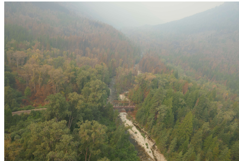
Photo 5: The CP Rail bridge across Cultus Creek.
