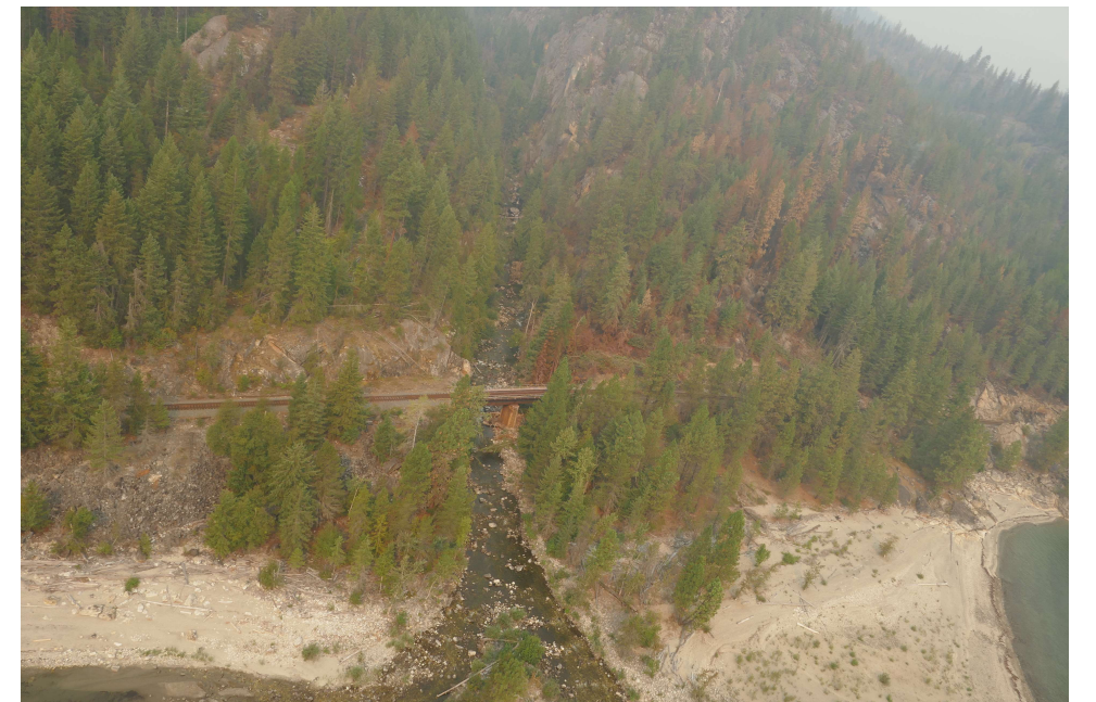
Photo 6: The CP Rail bridge across Next Creek.
